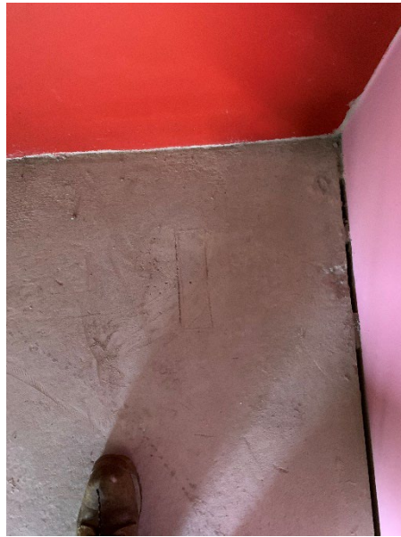
Top of landing showing grouted-in RVK hopper
