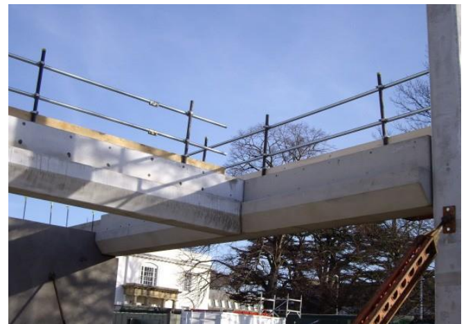
BSF connectors work equally well in beam/beam applications (as well as beam/column).
