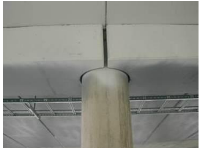
Corbel-less BSF design on round column.
