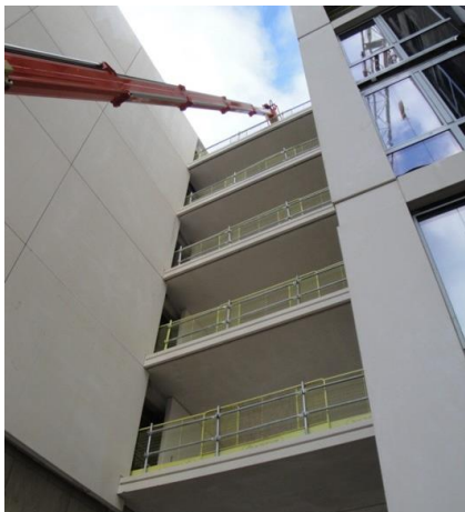
Floor units spanning considerable distance between structures
