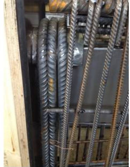
5.2 Beam unit inside the reinforcement cage
