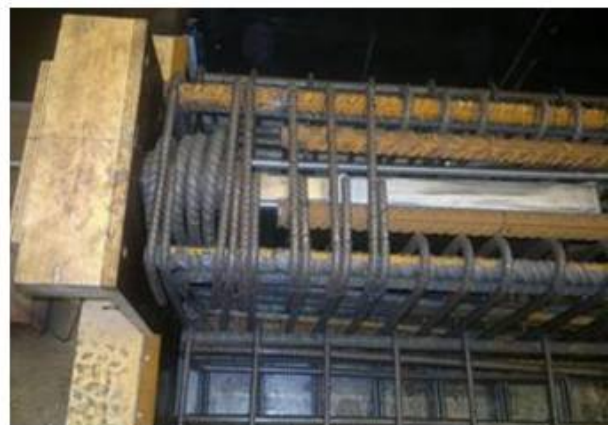
4.6 BSF-into final position in the form
