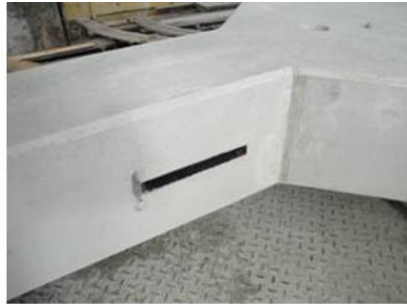
3.2 Finished column with BSF column unit
