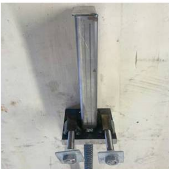
1.5 Column unit with threaded rods and plate washers
