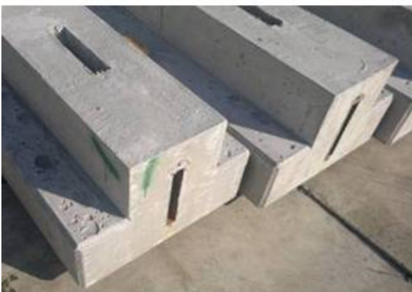
5.5 Inverted T-beam with BSF
