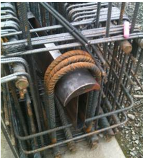
4.3 Beam unit inside the reinforcement cage
