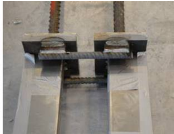
2.2 Column units welded together with reinforcement bar
