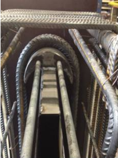
5.1 Beam unit inside the reinforcement cage
