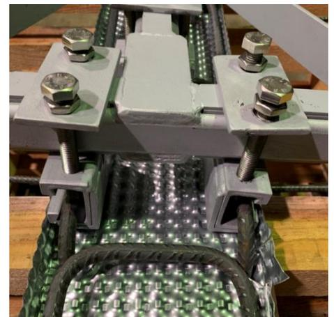
*Note: required casing edge distance to bars 20mm (usually 10mm) to allow tool access*
